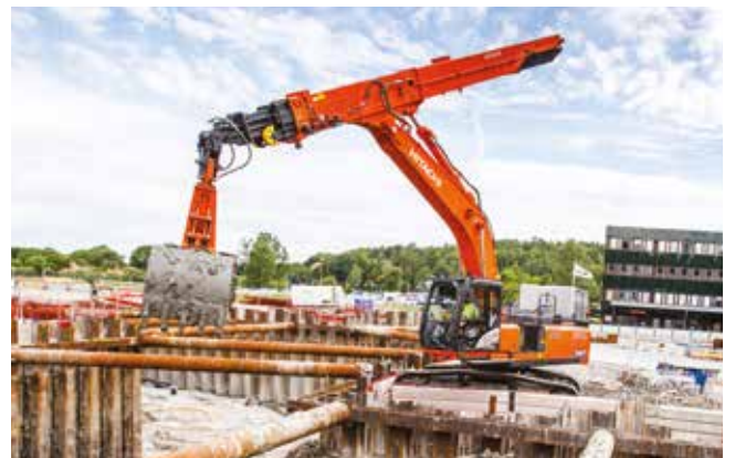
Special application excavators
