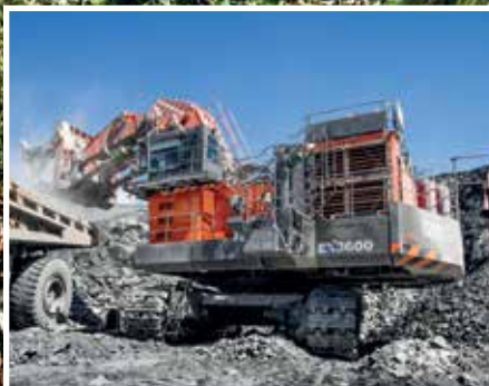
EX ultra-large excavators
